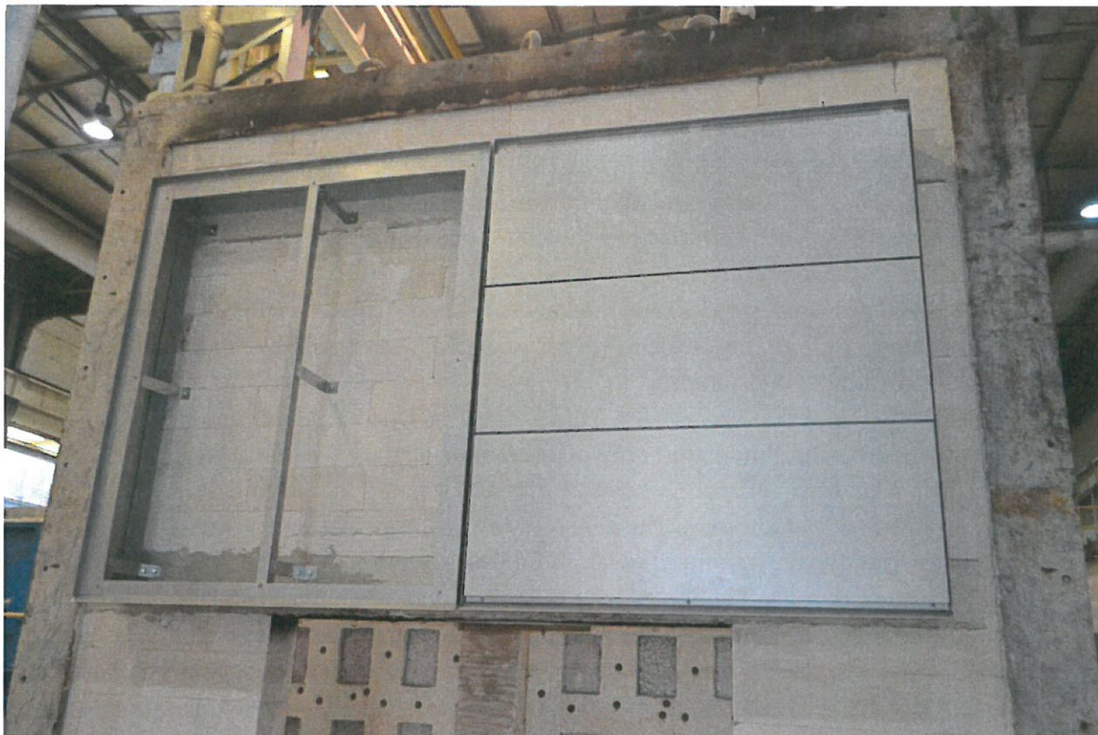
Fig. 27. Installation of the DEKMETAL façade
