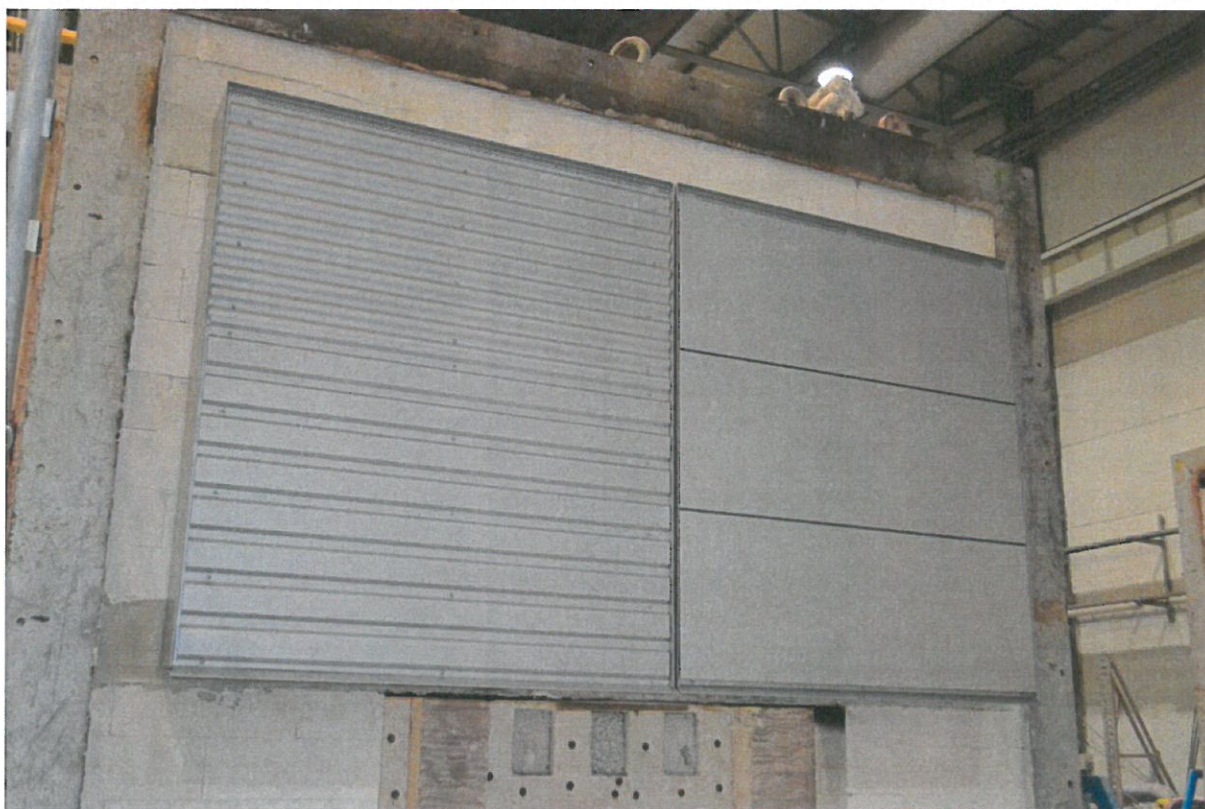
Fig. 28. Test specimen prior to the test
