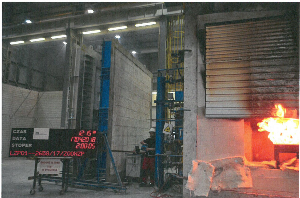
Fig. 40. Test specimen during the test t = 121 min
