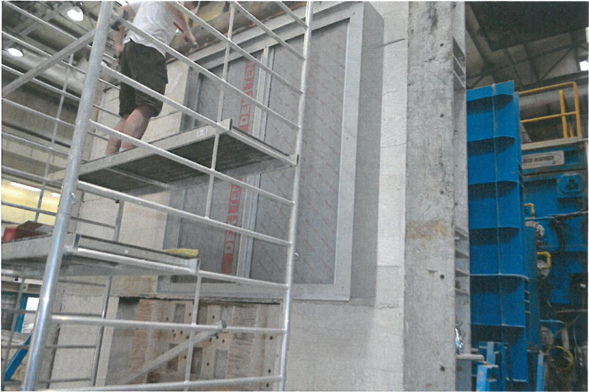
Fig. 25. Installation of the DEKMETAL façade
