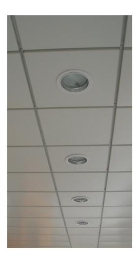
All ceiling parts can be made to measure with different sizes and shapes, which offers the customer large room for creativity. Apart from standard ceiling cassettes, our portfolio includes also variants of separately detachable cassettes for simple disassembly. A combination of various colours of color coated FeZn or Al sheet metal or use of STAINLESS STEEL with various types of finishes is possible.
