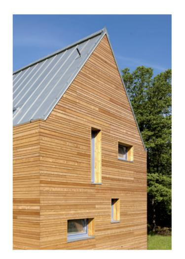
cross-section. It can have various sizes, materials (wood types), colours or surface finishes. They are usually not connected by any system of locks and every profile is separately attached to the steel substructure. For creation of a steel substructure it is possible to use a combination of DEKMETAL suspended supports and wooden battens (one-direction substructure) or a combined variant with DEKMETAL suspended supports, DEKMETAL metal profiles and wooden battens.
